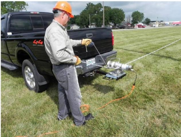
The Capstan hoist should be located between the operator and the load so the operator can maintain visual contact with both the Capstan load line and the material or equipment being lifted. However, if the hoist operator cannot be located in a position to view the load being moved, then communication with a second worker watching the load is necessary. Proper communication and signals must be used between crew members when lifting is occurring.
